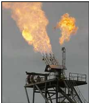
POSEIDON flare with water injection.
