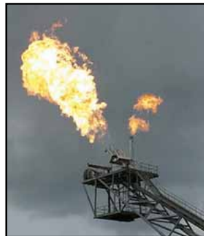
POSEIDON flare without water injection.
